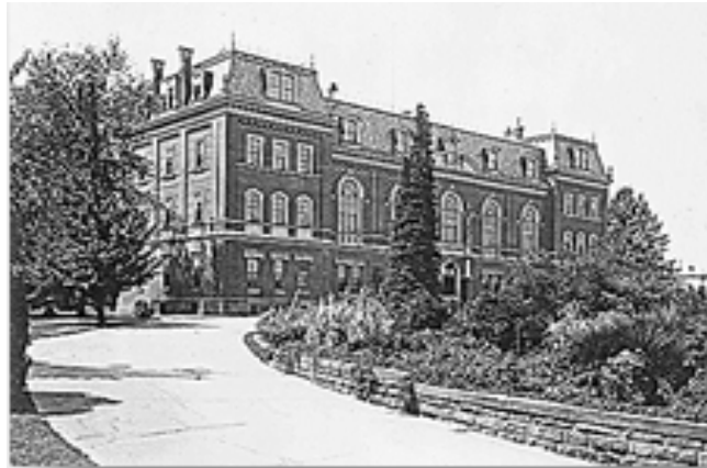
Figure 13: USDA Administrative Building, 1917
